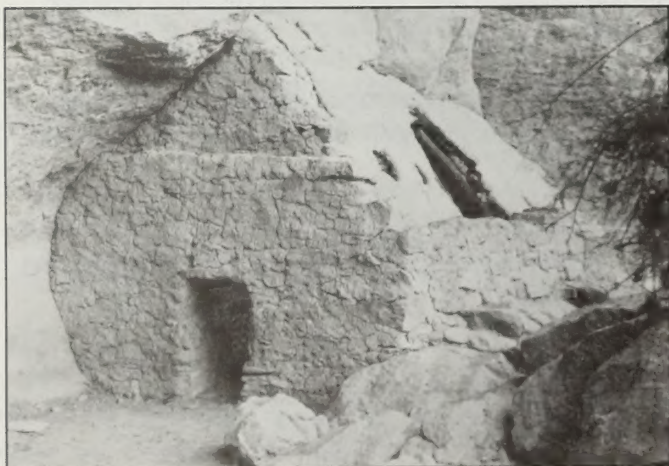
The Turkey Creek cliff dwelling is one of the most intact prehistoric structures of its kind in southeastern Arizona.
